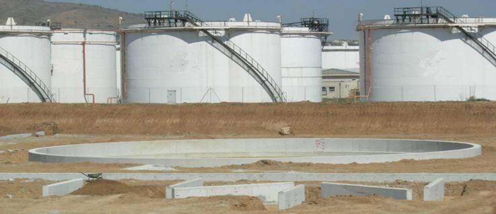
Kırıkkale Refinery Sulphure Removal Unit Construction, Tank Farms/Turkey/2005 Client : TÜPRAŞ
